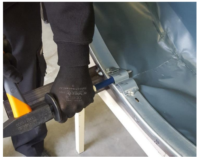
Figure 24. Hammer it underneath the clamping clip
