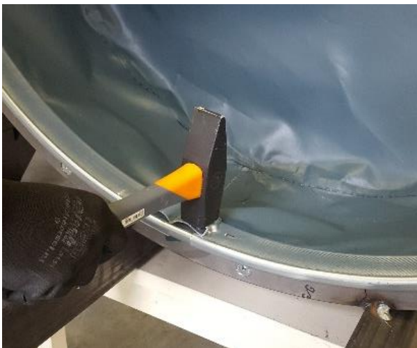
Figure 21. Repeat until the Clamping Clip is flat
