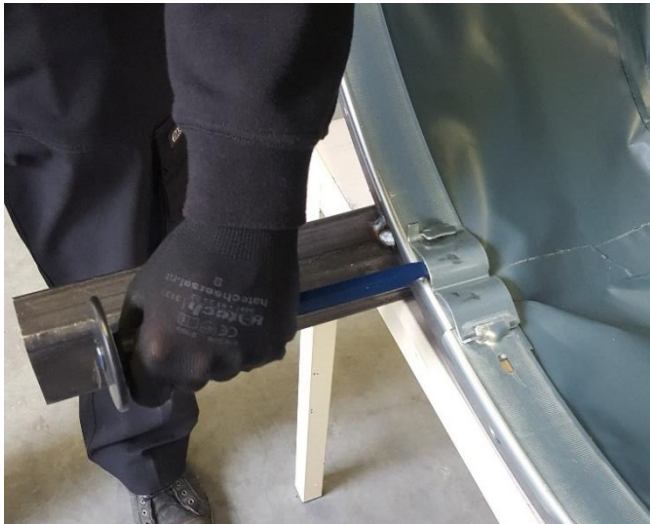
Figure 23. Place the chisel
