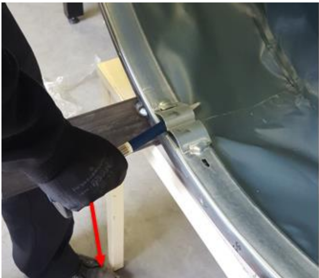
Figure 25. Push the chisel downwards
