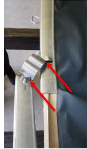
Figure 12. Place Clamping Clip diagonally
