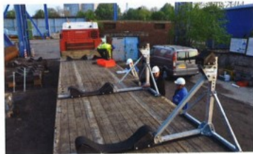
Figure 7. Pipe Raiser assembly finished.
