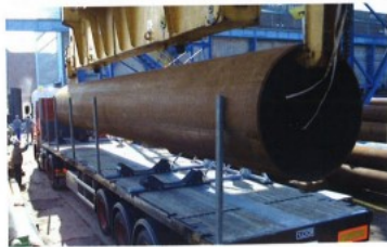
Figure 8. Loading the first pipe.
